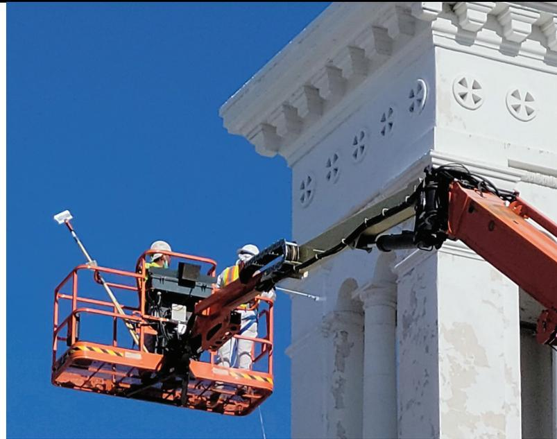
Determined to get the job done, Dougall estimated he needed a 150' boom lift, but a 185' lift was the only one available. The job required barricade permits from the city because the lift would occupy three lanes of an adjacent street. The city quickly complied, and Desert View's four-man crew persevered. They pressure washed and scraped the tower walls, applied two coats of a custom-formulated elastomeric primer, and then two coats of EVERSHIELD® Ultra-Premium Exterior Flat Paint in white.
